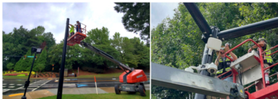
Ouster digital lidar deployment on a traffic intersection (Photo: Business Wire)
